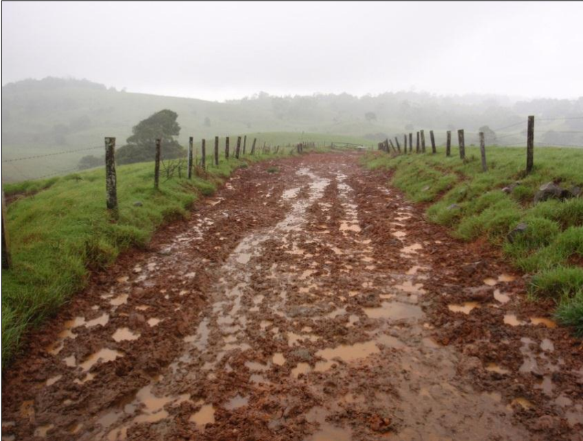
Left: The western laneway prior to the project. The laneway has eroded to the point where it traps and holds water resulting in an excessively boggy surface.
