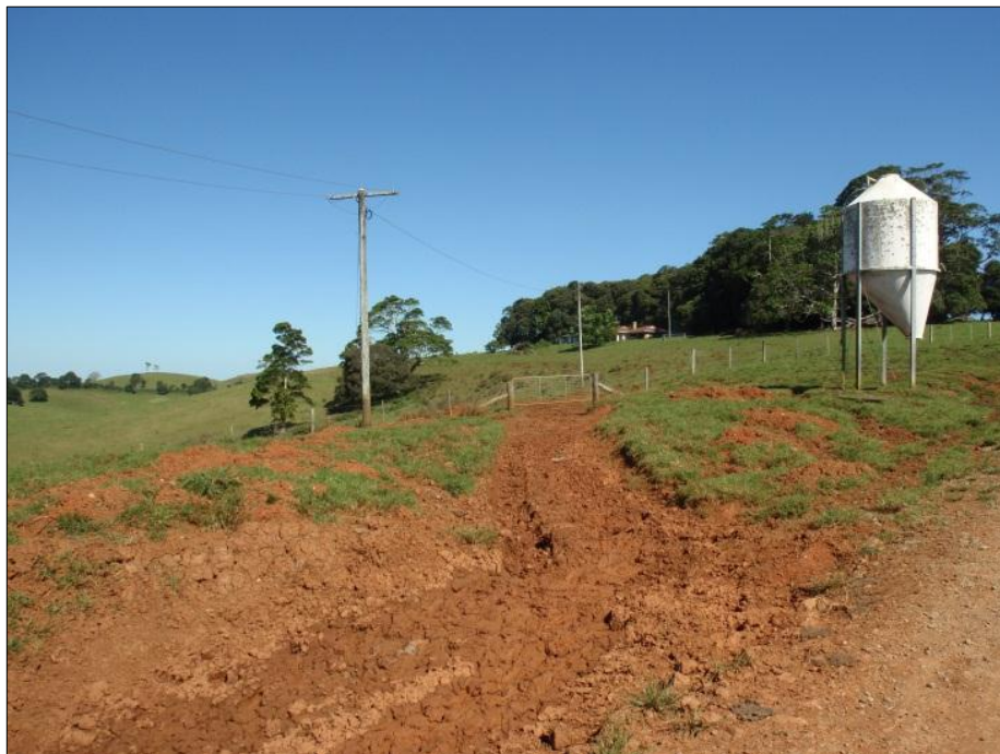
Left: The eastern laneway from the dairy entry road prior to works. Note the poor drainage.
