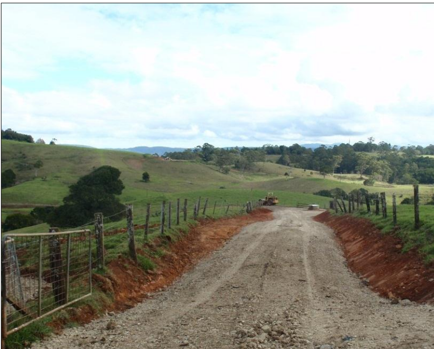
Left: The western laneway profiled and hardening to create a free draining durable surface.
