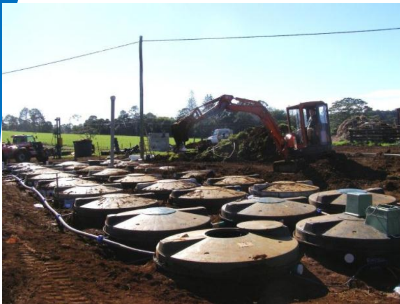
Installation of Biolytix wastewater treatment system
